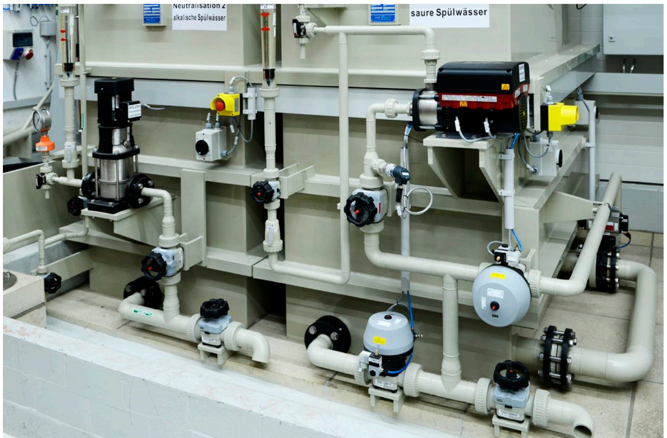
Fig. 1: Industrial wastewater treatment will become more important in the future, as shown here in a neutralization plant for wastewater in surface coating
